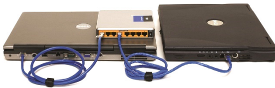
A switch connected by UTP cable to two PCs
